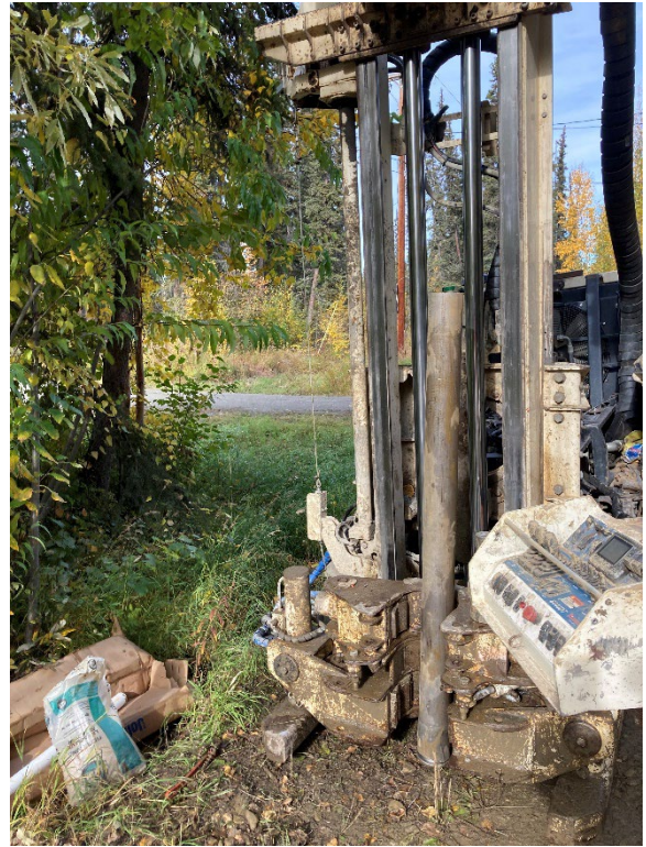
Exhibit 2-1: GeoProbe 8040 DT setting a monitoring well using 4-inch dual core
